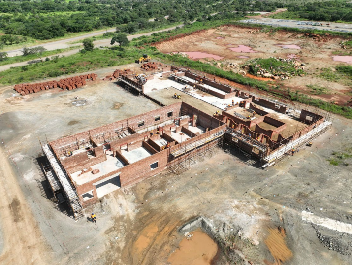
Laboratory Brickwork Construction
