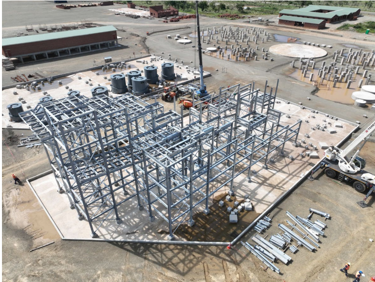
Cleaner Flotation Steel Erection
