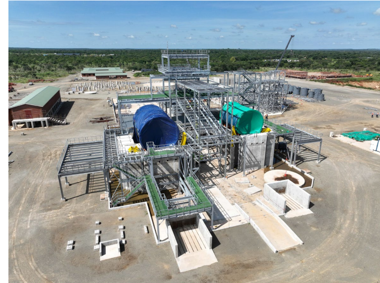
Mill Building Steel Erection
