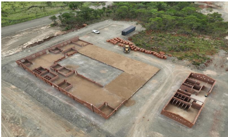
Civil construction progress (Admin building)
